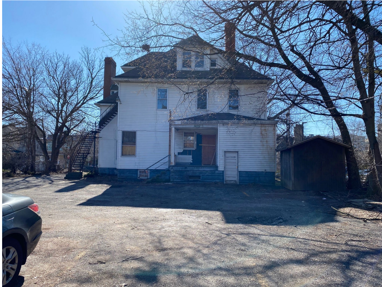
REAR (NORTH) FACADE
