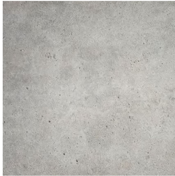
Cast in place concrete foundation
