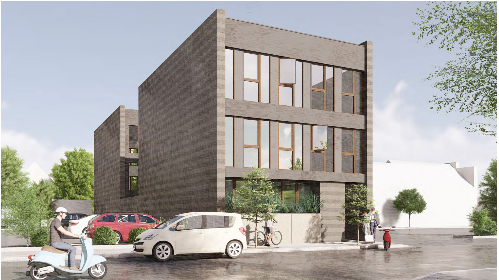
View 2 View looking at east and south facades
