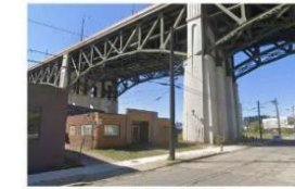
4 WEST 3RD STREET LOOKING NORTH WEST
