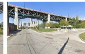
2 WEST 3RD STREET LOOKING NORTH
