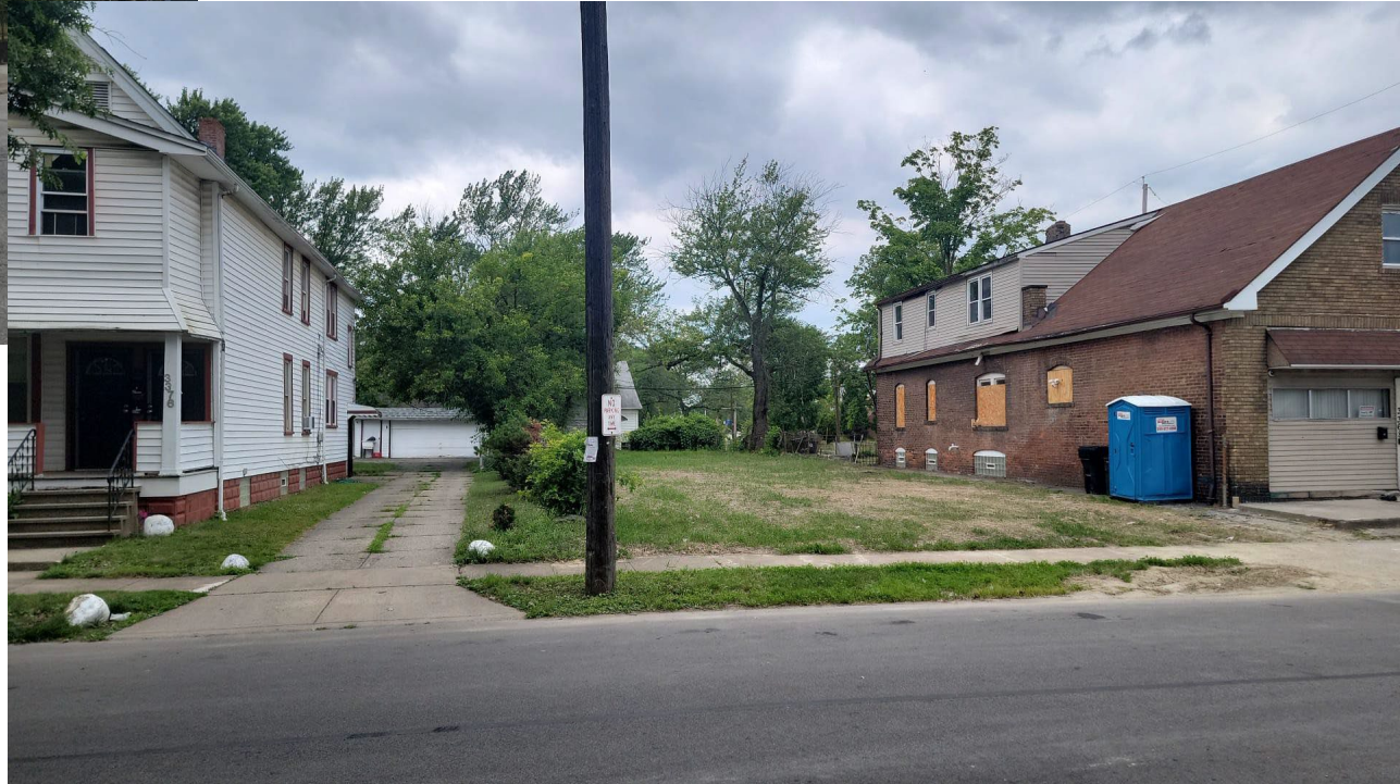
Left side of building
