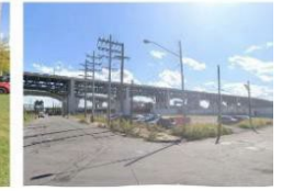
7 WEST 3RD STREET LOOKING NORTH WEST
