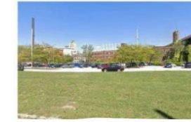
9 WEST 3RD STREET LOOKING NORTH WEST
