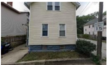
STREET SIDE PHOTO 6
