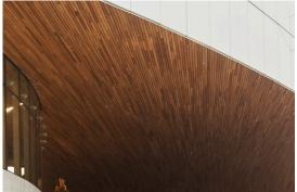
Metal panel soffit with wood grain texture and finish
