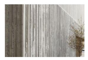
Concrete with architectural formwork finish and light gray integral color
