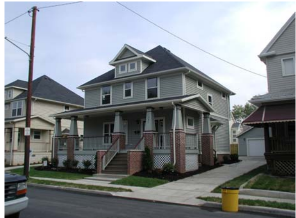
Citirama 2004 in Glenville neighborhood offers diverse architectural styles, while maintaining the unique character of the neighborhood.
