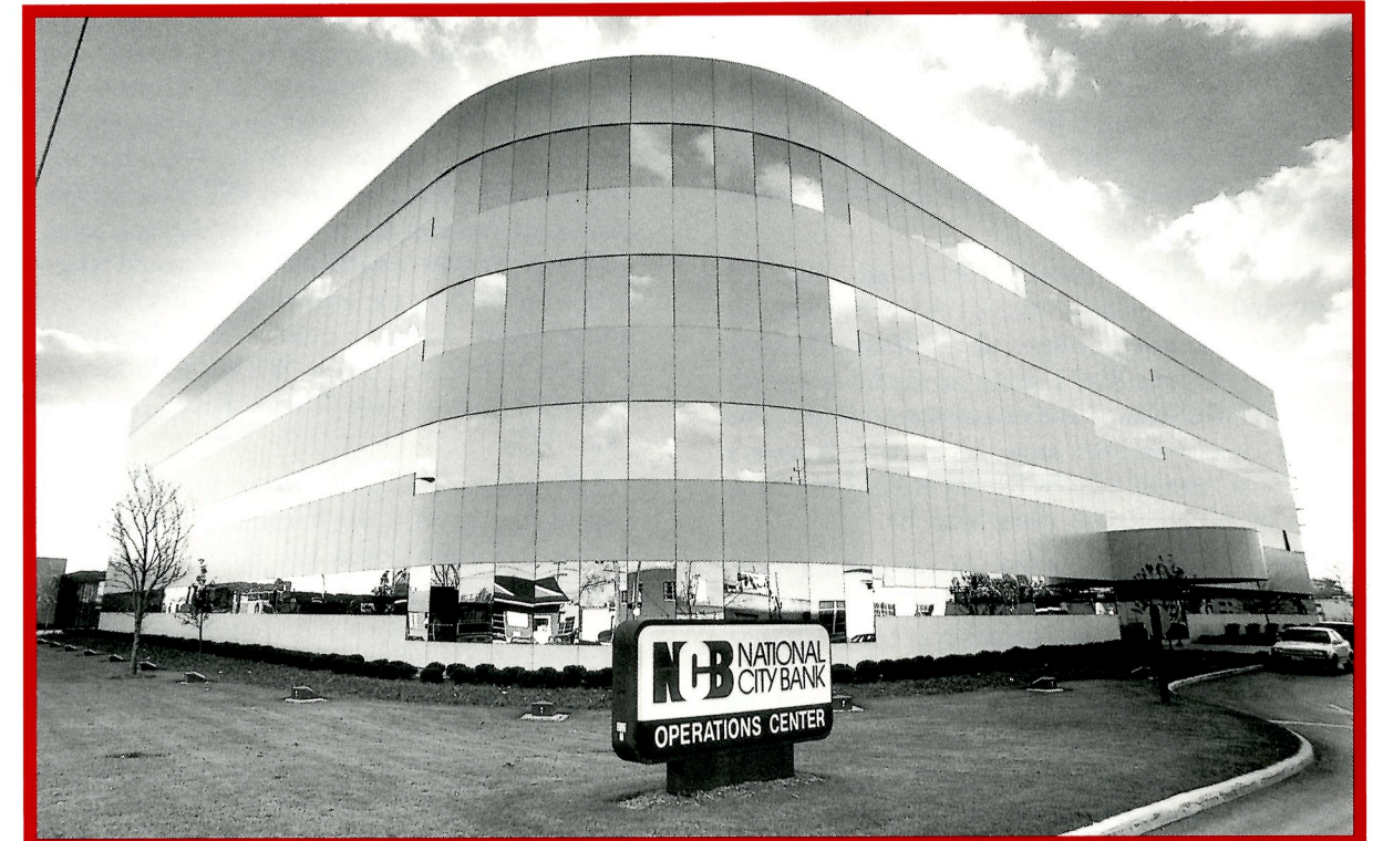
The potential for office development in proximity to freeway interchanges in Cleveland is demonstrated by the presence of a major bank operations center at the West 150th Street interchange of I-71.
