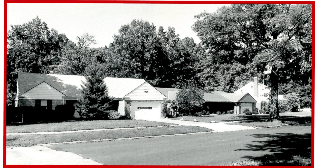
The greatest concentration of suburban-style housing in Cleveland is found in the West Park neighborhood. (LOCATION: West 159th and Edgecliff).
