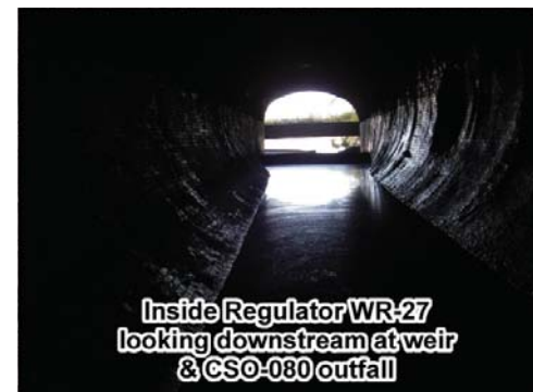
Walworth Run is currently culverted all along Train Avenue in this combined sewer outfall.
