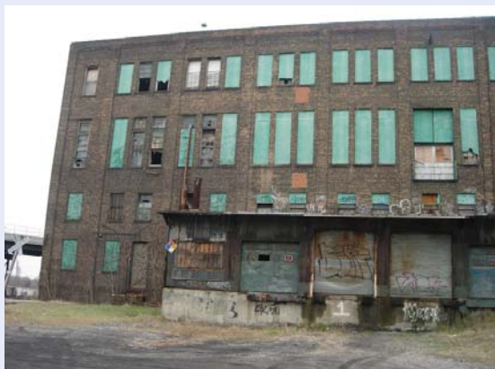
All around Cleveland dying or weakened industries leave behind graveyards of underutilized or vacant buildings. This building along Train Avenue was at one point a thriving brewery.
