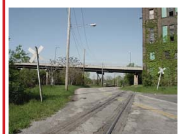
Railroad tracks cross road and Train Avenue All-Purpose Trail. Appropriate crossing signage needed.
