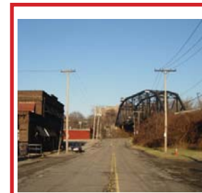
Train Avenue All-Purpose Trail jogs from the North side of Train Avenue to the South side, with one street crossing.
