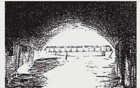
Walworth Run was culverted in a combined sewer overflow.
