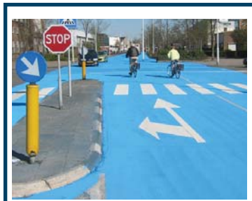
Train Avenue All-Purpose Trail changes color to represent Walworth Run and Mill Pond past presence.
