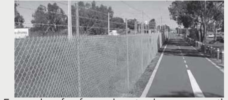
Example of a fence barrier between trail & rail
