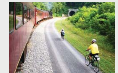
Example of no barrier between rail & trail Great Allegheny Passage, PA & MD
