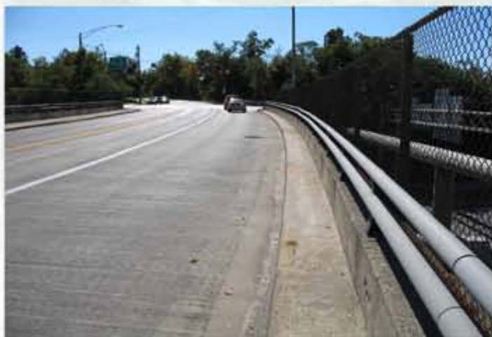
Where Rocky River Drive / Riverside Drive bridge over I-90.
