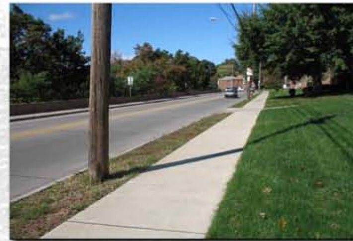
Unmarked pavement on Rocky River drive / Riverside drive.
