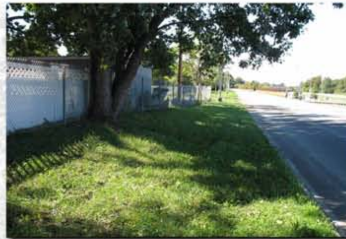
Tight space between existing property lines and South Marginal.
