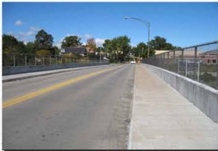
A typical narrow bridge that spans I-90
